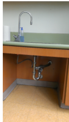
Typical classroom sink without bubbler
