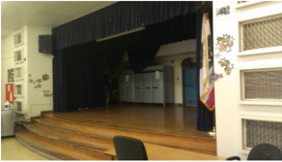
Aged Cafeteria/MPR diffusers
