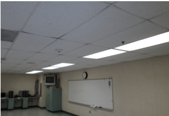
Typical condition of interior recessed light fixtures
