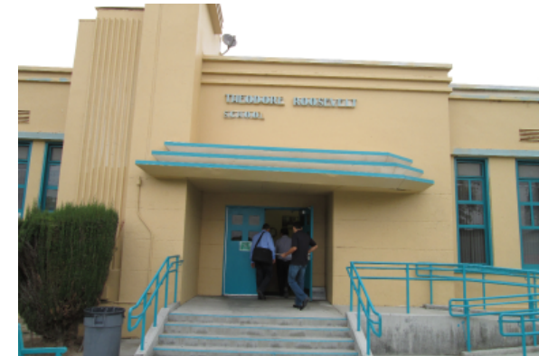
Lack of security cameras
