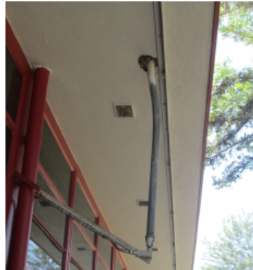
Unsafe installation of light fixture conduit
