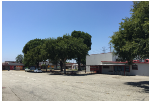
Inadequate site lighting coverage
