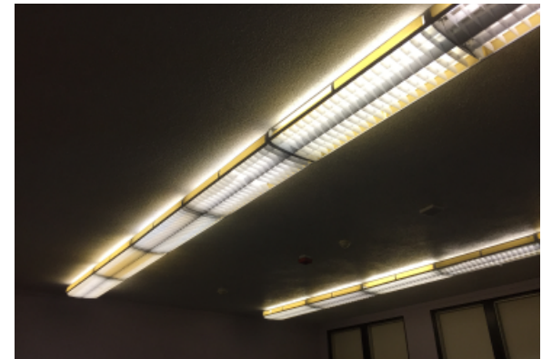
typical condition of interior surface mounted light fixtures
