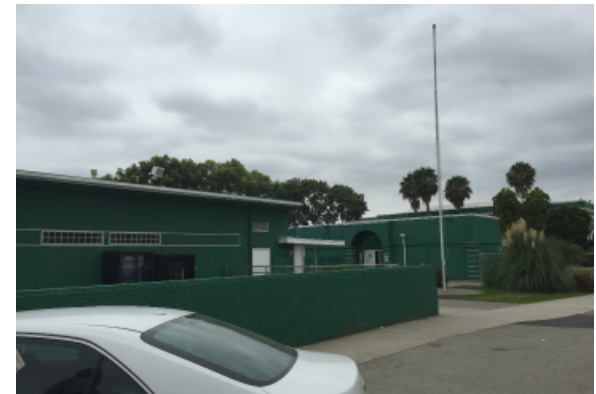
Lack of security cameras
