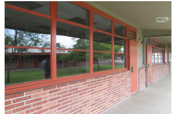
Typical single pane windows
