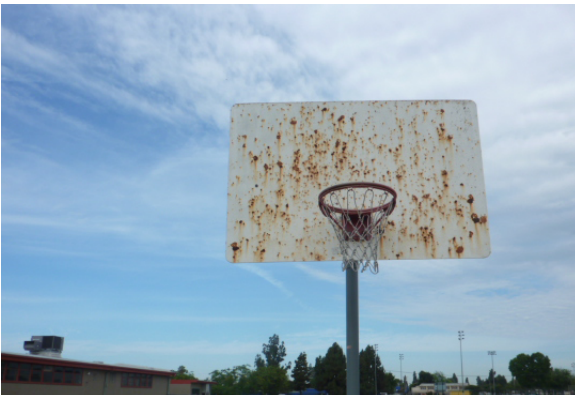
Degraded backboard on playground
