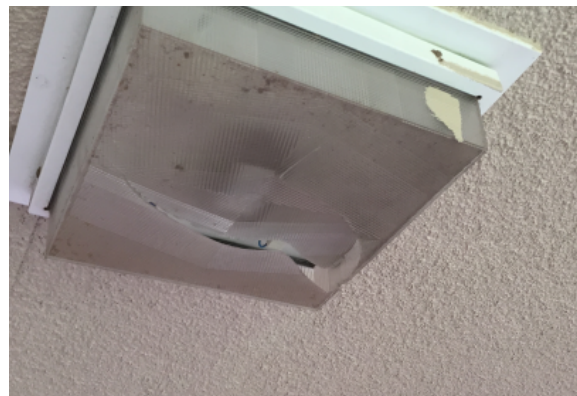
Typical condition of exterior surface mounted light fixtures
