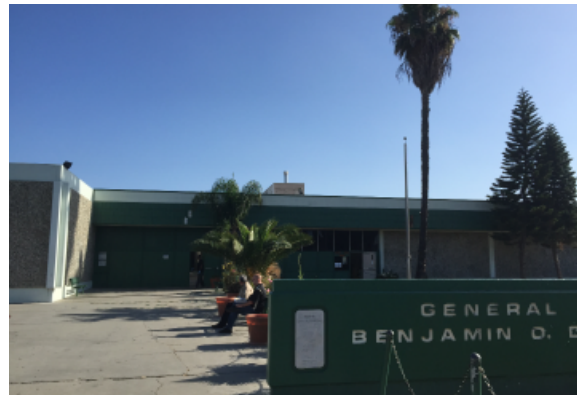
Lack of security cameras
