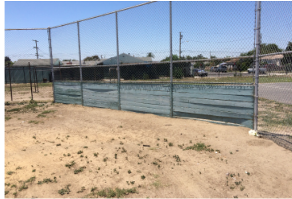
Backstop is broken/rusted, no landscape
