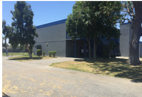
2-story modular classroom building(2004)
