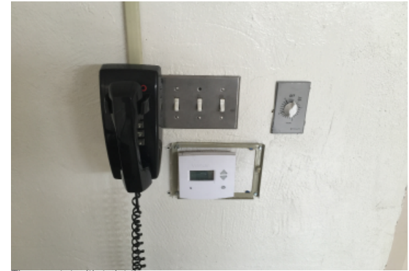
Thermostat with twist timer
