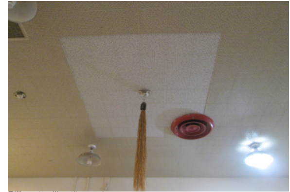
Different ceiling tile repair
