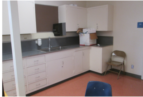
Original casework and sink not accessible
