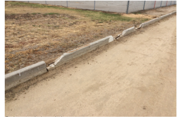
Curb on track degraded
