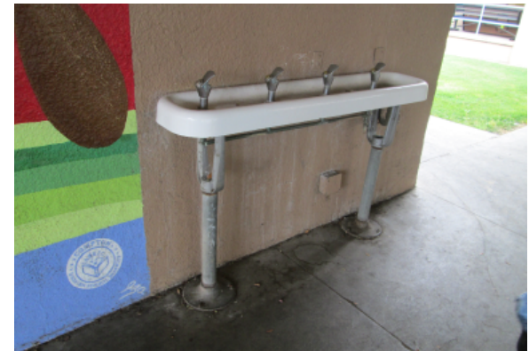
Non ADA complaint drinking fountain
