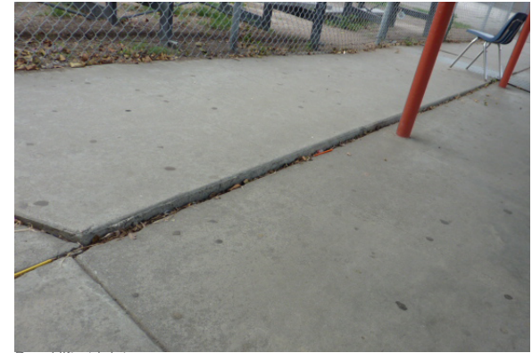
Panel lift at joints
