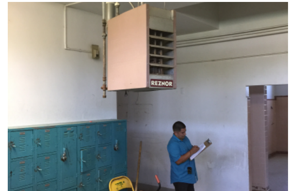
Nonfunctional locker room floor drain
