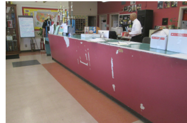
Non ADA complaint administration counter
