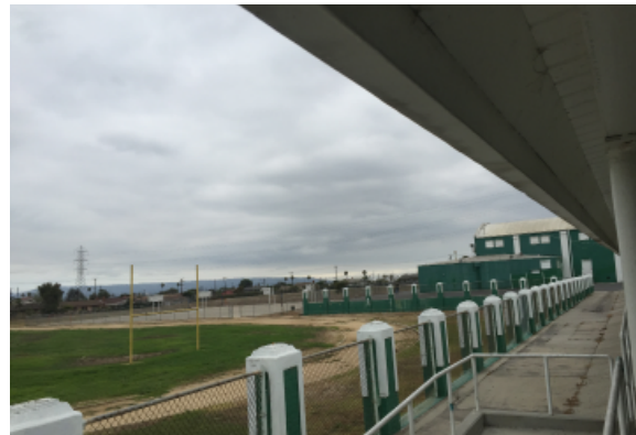
Inadequate site lighting coverage
