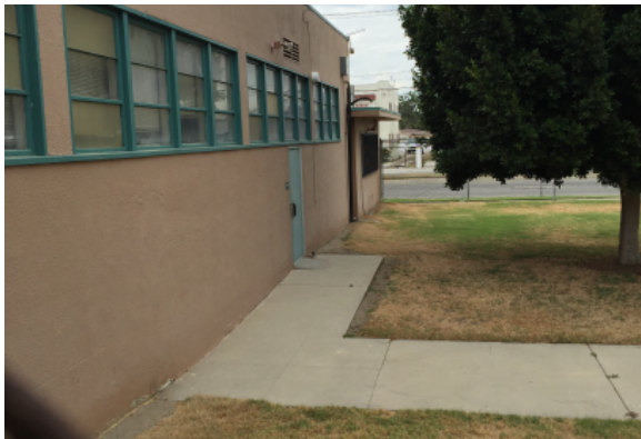
Lack of security cameras
