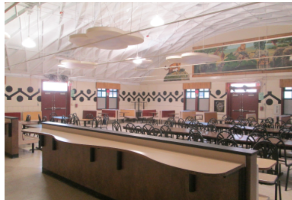
Non ADA complaint counters
