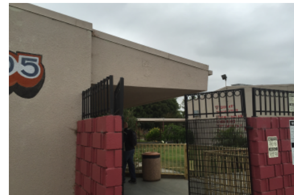
Lack of security cameras
