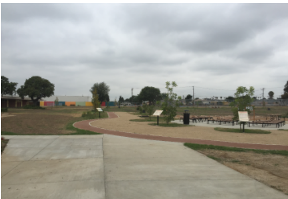
Inadequate site lighting coverage
