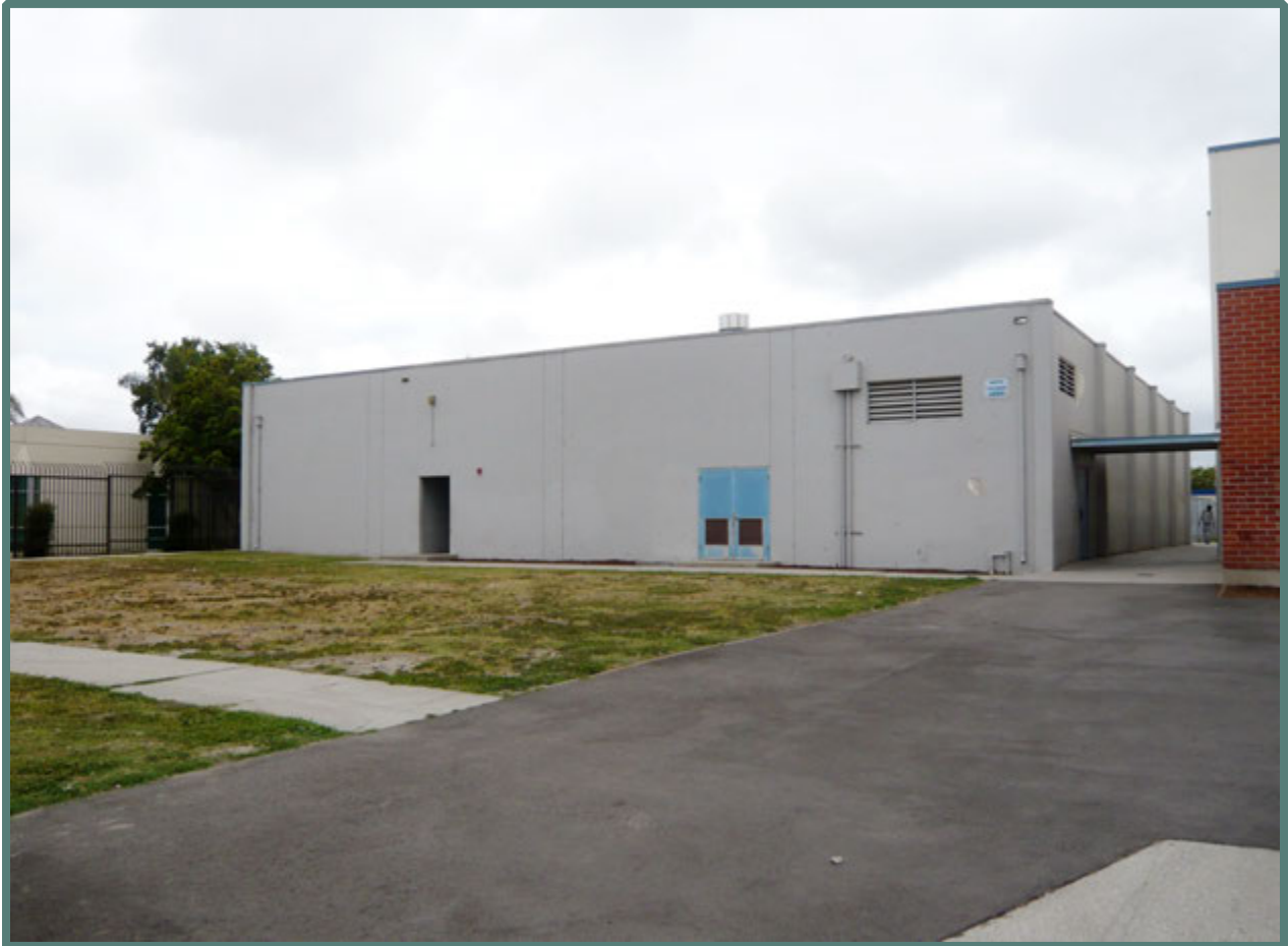
BUILDING "M-2" GIRL'S LOCKER ROOM
