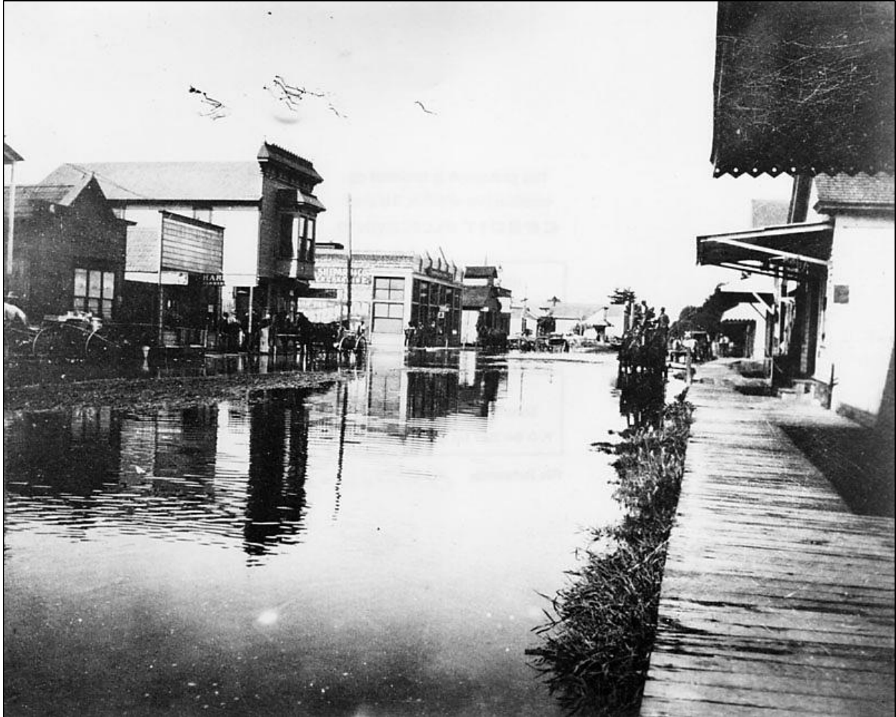
Figure 14. View of flooded Streets in Compton looking west on Compton and North on Alameda. (Photo courtesy of Los Angeles Public Library Unique Identifier 00020473.
