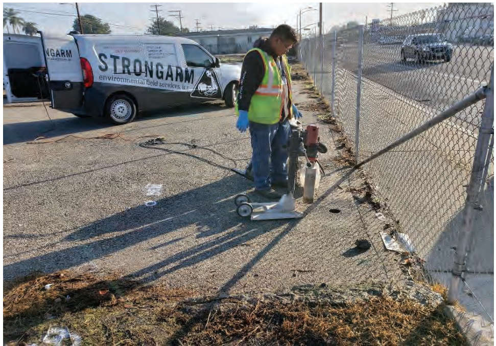
Photograph 28: Worker positioning a corer to drill through asphalt on AOC5.
