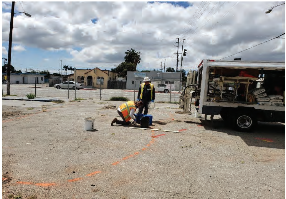
Photograph 26: Workers installing soil vapor probes on AOC4.
