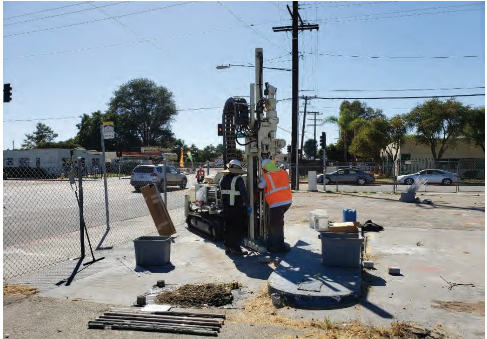
Photograph 27: Workers using a 6620DT direct push rig on AOC4.
