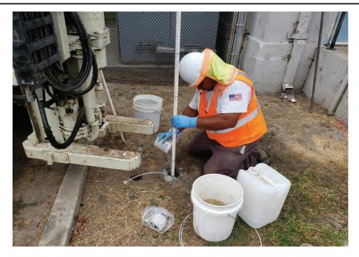
Photograph 13: Soil Vapor probes being installed at AOC3-B1 on Compton High School main campus.
