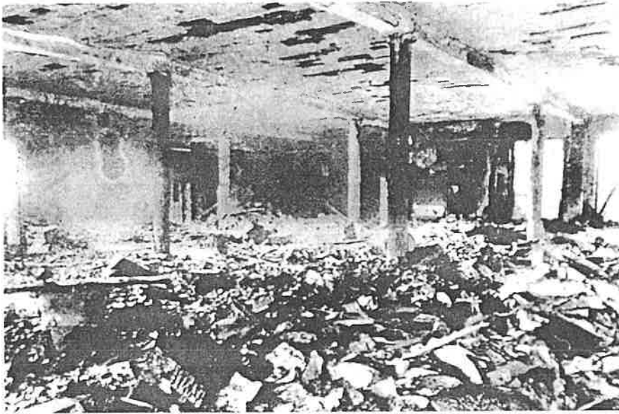
This is a photograph of the gutted tenth floor of the Asch Building that was taken in the aftermath of the fire.
